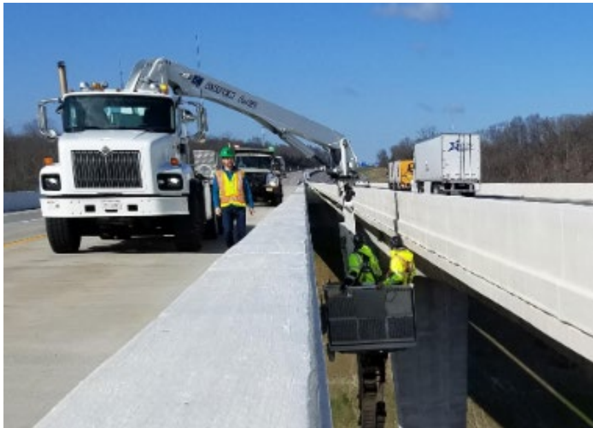
Attaching Fiber Optic Cable to Existing Bridge
