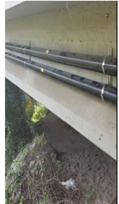
Fiber Optic Cable Attached to Existing Bridge
