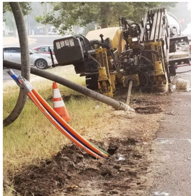
Horizontal Drilling Rig and Conduit
